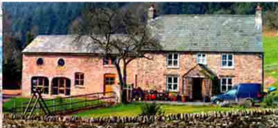
First group of buildings at the South end of the reservoir.
